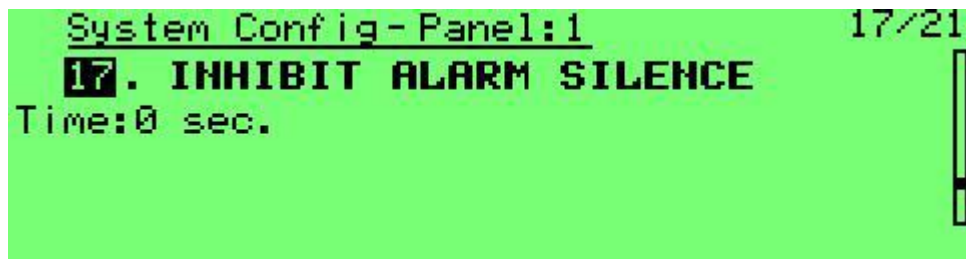
Screen 62 System configuration – inhibit alarm silence
